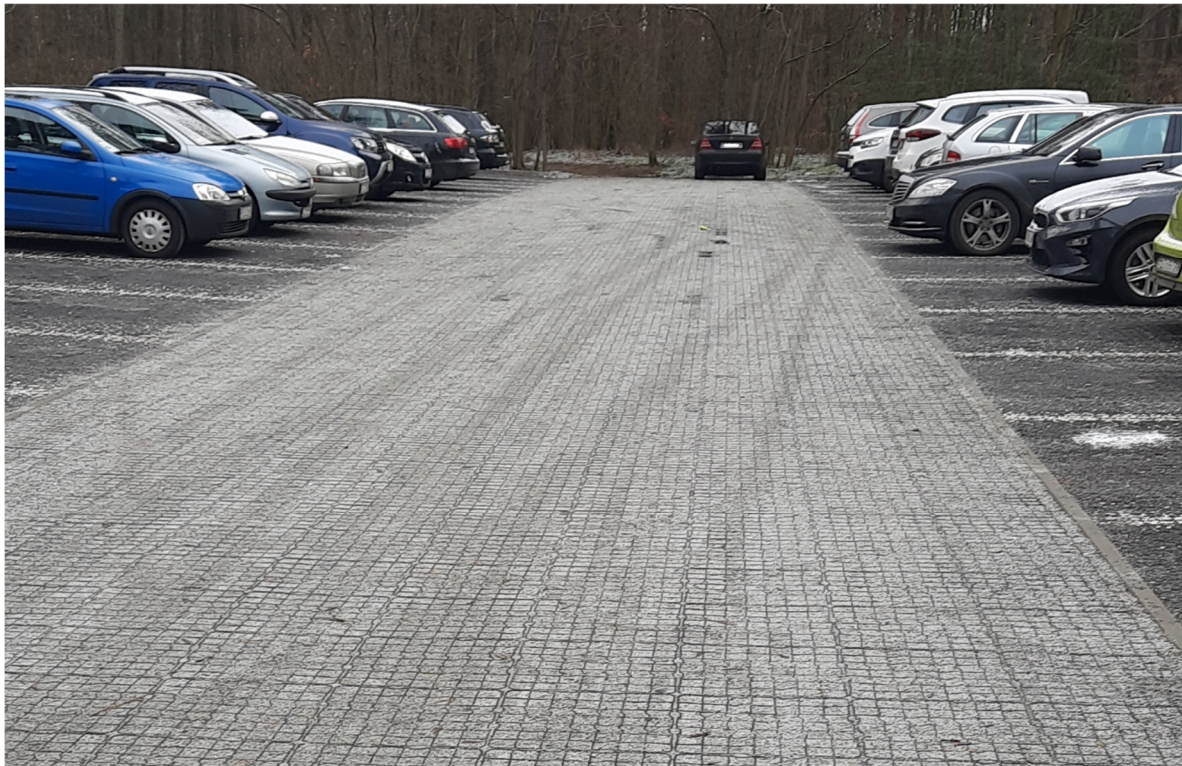
Figure 2. Example of rainwater permeable parking places and manoeuvring area—Zielona Góra, Cisowa Street.
