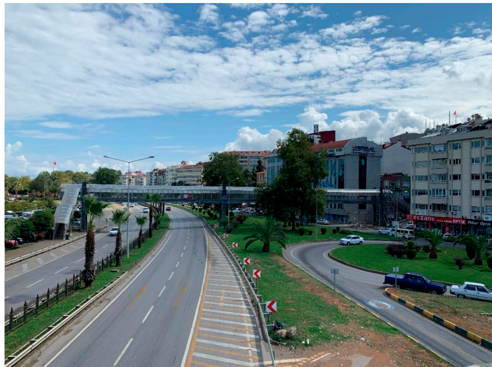
Figure 2. The view of the overpass over the road no. D010, also known as the Black Sea Coastal Highway, after construction of the roofing. Source: own study.
