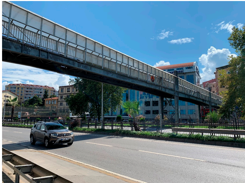
Figure 3. The view of the overpass over the road no. D010, also known as the Black Sea Coastal Highway, after construction of the roofing. Source: own study.
