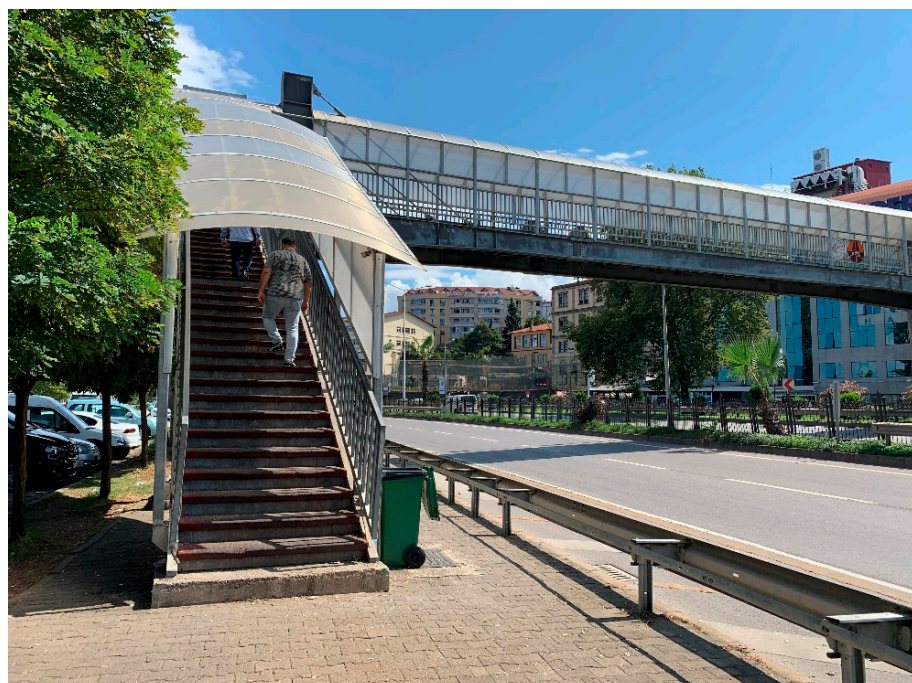
Figure 8. The overpass suspended over the highway no. D010 after constructing the roofing.
