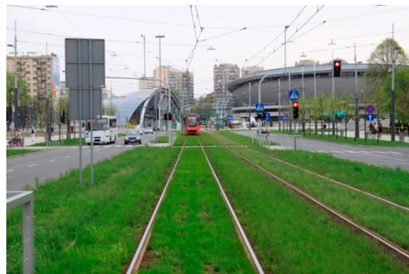
Figure 4. Poland, Katowice, W. Grassy tram lane along Kofranty Avenue. Photo: B. Fortuna-Antoszkiewicz, IV 2016.
