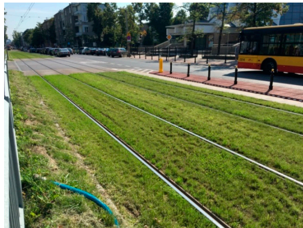
Figure 16. Warsaw: Rakowiecka Street, Mokotów district. The grassy track cover after mowing during summer. Photo: J. Łukaszewicz, VIII 2016 [65].
