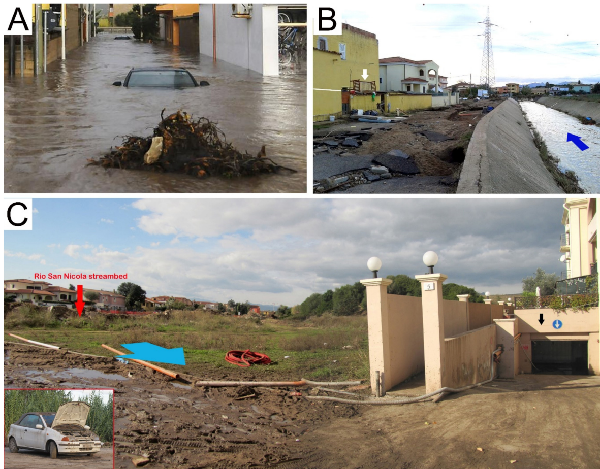
Figure 9. (A) Olbia: Although about 15 h had passed since the paroxysmal phase, in some morphologically depressed areas of the city the water remained well above 1.3–1.4 m in height. Some cars were totally submerged in one of the streets most affected by the flood in the Baratta quarter (courtesy of private citizen). (B) Olbia, left bank of the Rio Seligheddu Stream, canalized stretch (foto Luino). Water level left a marker on the wall, which is evidenced by white line. The height of the waters is evidenced by the bed dragged and placed over the roof of the ground floor (white arrow). (C) Olbia: very common situation along the areas close to the streambeds (foto Luino). In this image, the Rio San Nicola (red arrow) waters exceeded the natural bank that was devoid of embankments or retaining walls and easily reached the houses located on the left bank, which was a short distance away. In many houses, the underground garages have been foolishly built and had been totally flooded (black arrow indicates the level), with serious damage inducted to parked cars. The extracted cars are so saturated with fine material (silt and clay) that they had to be demolished (image in the left corner).
