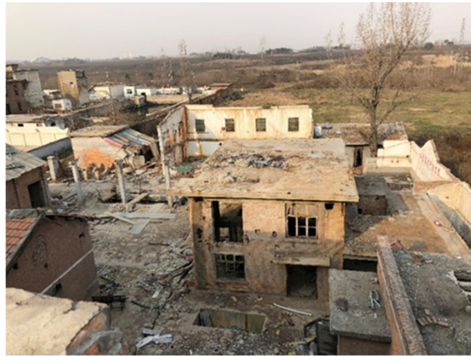
Figure 7. Abandoned factory site of the Jiaoda Ruisen chemical plant in the study area.
