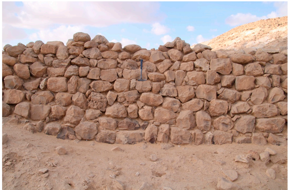
Figure 9. Type B agricultural terrace in the Negev Highlands. Note the collection of building stones used for the construction, composed of limestone and chert collected and quarried slabs. The uneven collection of stones in the middle can hint at occasional collapse and restoration during the cultivation time. (Photograph: Y. Avni).
