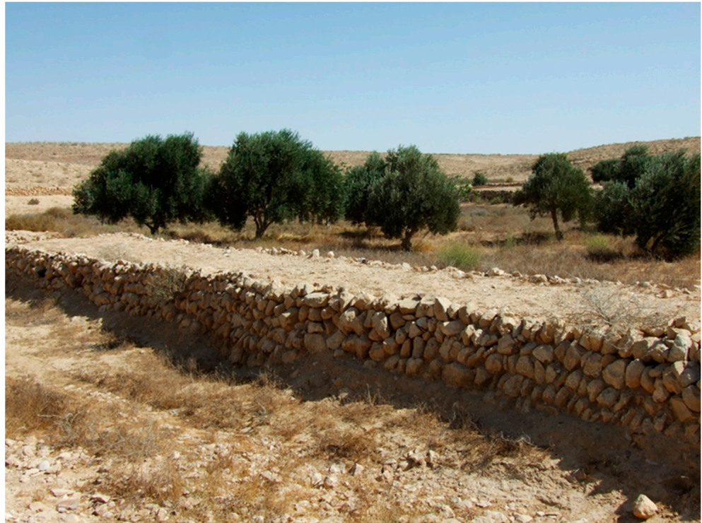
Figure 8. A reconstructed Type B agricultural terrace in the Negev Highlands designated for the cultivation of perennial plants, such as olive trees and vineyards. (Photograph: Y. Avni).
