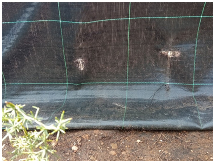
Figure 7. Large holes on the geotextile caused by wild boars.
