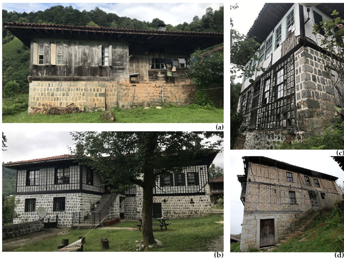
Figure 5. (a) Timber buildings elevated on stone in Hara village; (b) stone-infilled building in Çağlayan village; and (c) mixed construction on a building in Hara village. The stone and stone-infilled technique on the ground floor and the plastered façade of the first floor is an example of the çakatura technique. Source: Photograph by the first author taken in July 2019. (d) Amulet-filled building in the district of Pazar in Rize. Source: https://karadeniz.gov.tr//konut-ahmet-sakir-efendi-konagi/#prettyPhoto (accessed on 8 February 2022).
