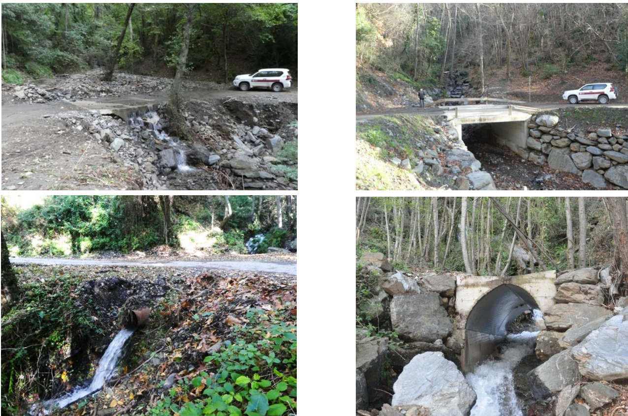
Figure 14. Modified bridges to recover the natural stream bed and to allow the displacement of aquatic fauna along them. Left images: before recovering structure. Right images: the same locality after recovering structure.
