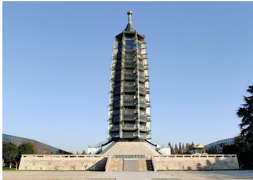
Figure 7. The overall appearance of the rebuilt Porcelain Tower (Source: photo courtesy of Pengfei Ma).
