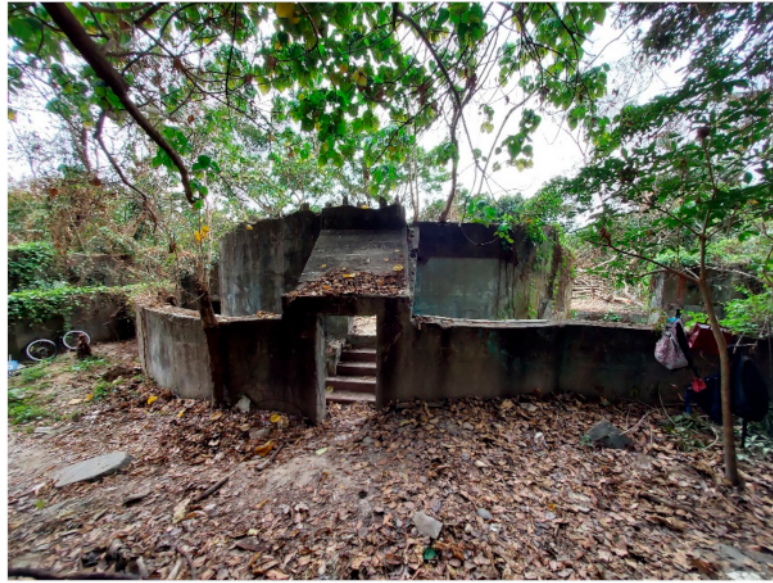
Figure 6. Gun Emplacement 1 of Jubilee Battery within the University of Chicago Hong Kong campus—in ruins (after clearance by volunteers) in March 2021.
