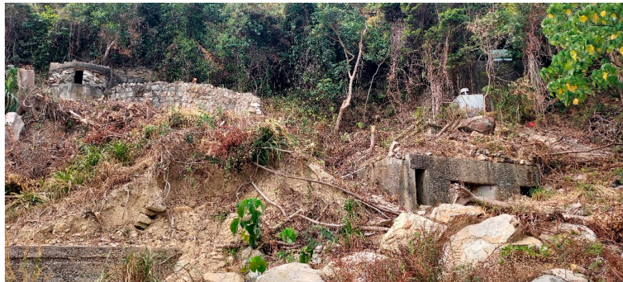
Figure 1. Pillbox 14 and its search light shelter cleared by volunteers before squatting (May 2021).
