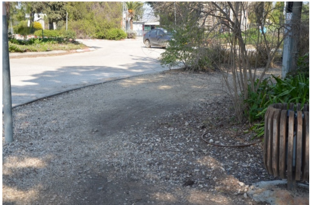
Figure 16. Missing sidewalk in Nahalal. Photo by the authors.
