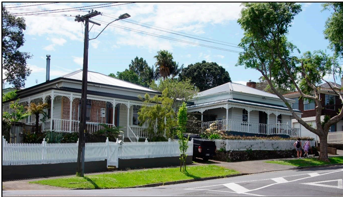
Figure 4. Normans Hill Road, Onehunga (Authors' photograph, September 2020).
