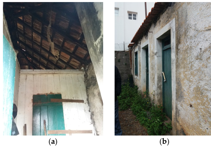
Figure 3. Building incompatible with residential use in the parish of Caniçal: (a) damaged roof; (b) main door.
