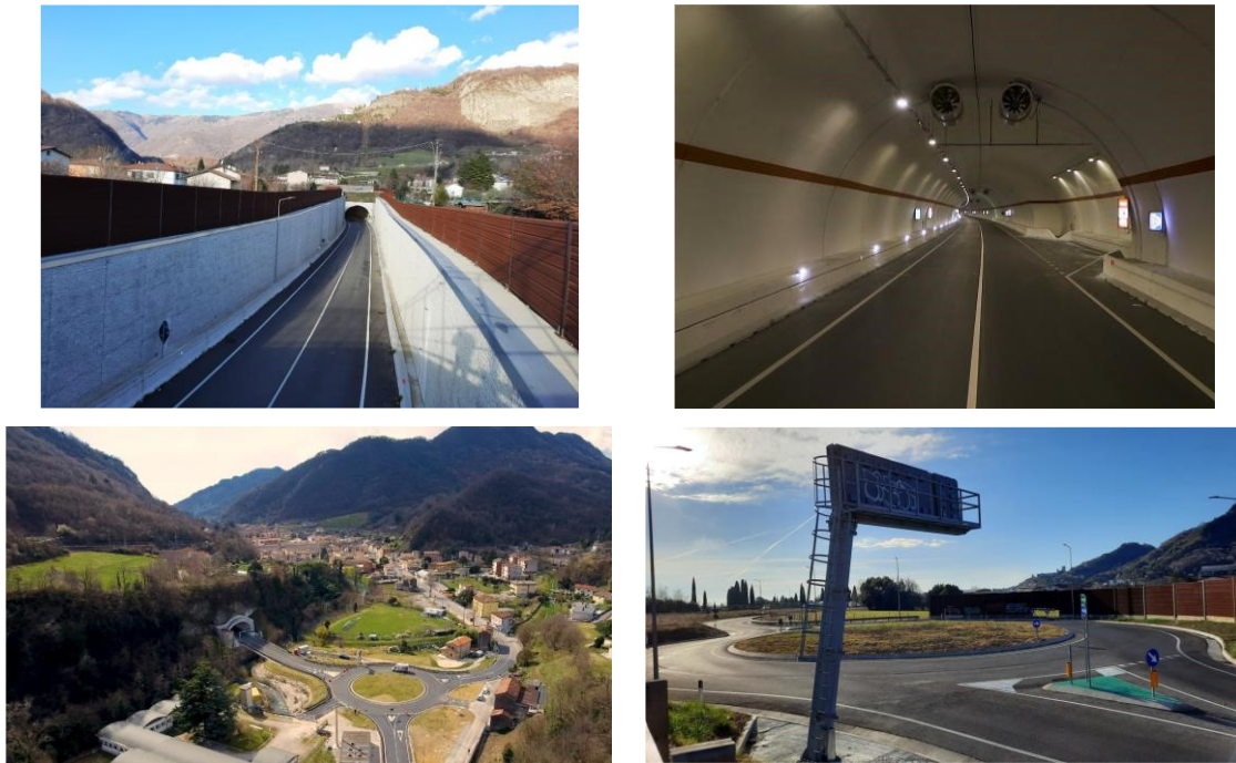
Figure 3. Project picture after completion in 2021.
