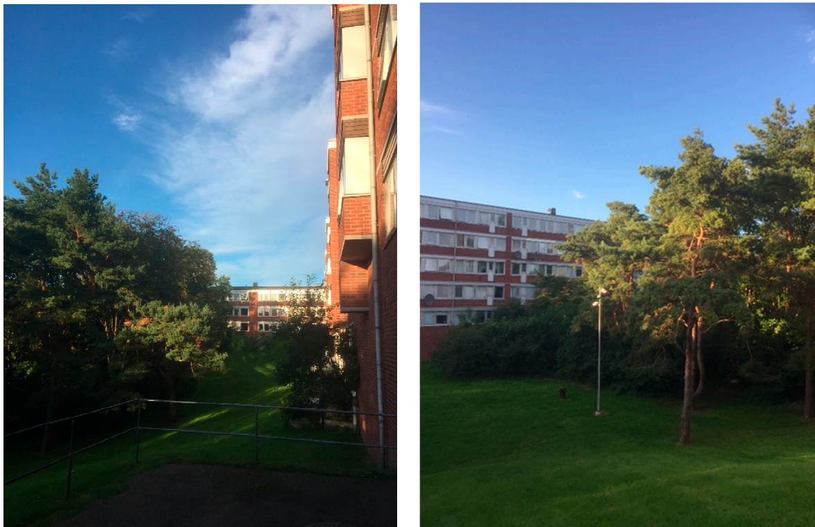
Figure 9. The inner yard of 164:14 is on a steep slope and dominated by trees.
