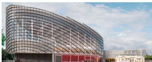
Figure 9. Concentric circle geometry projection on complex building facade surface generates solar shading tubular element pattern. Source: Tzortzi, Visconti, [22].
