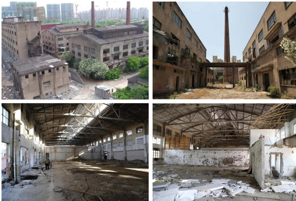
Figure 1. (top left): Original view of Shanghai Nippon Sanitary Bottle Factory. (top right): Big chimney in the site. (bottom left): Big space without columns and high ceiling. (bottom right): Original view of the interior space of the factory. Source: https://m.thepaper.cn/newsDetail_forward_14466796 (accessed on 10 November 2023).
