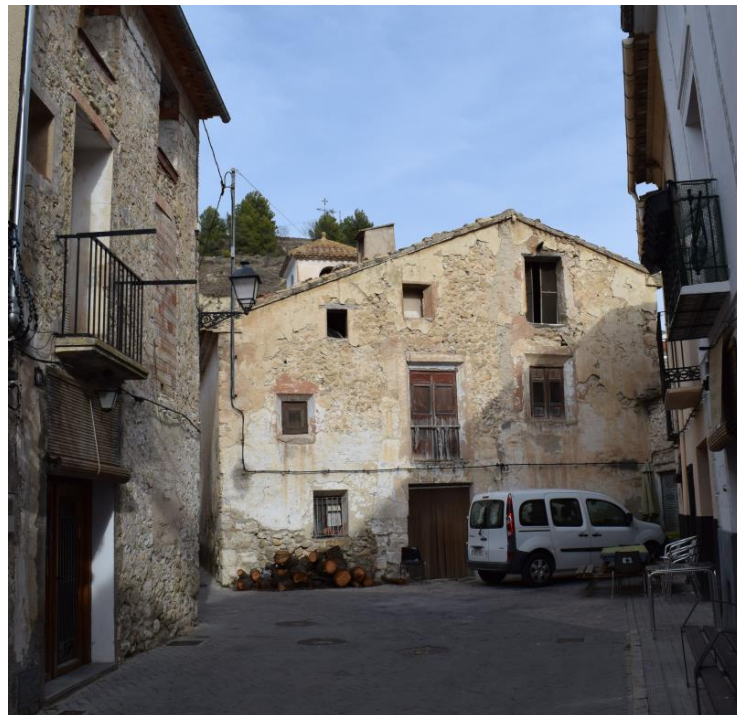
Figure 12. Vernacular dwelling in a poor state of conservation located on Calle de la Iglesia, Ares del Bosque, Benasau, 2024. Author: Eva Tortajada.
