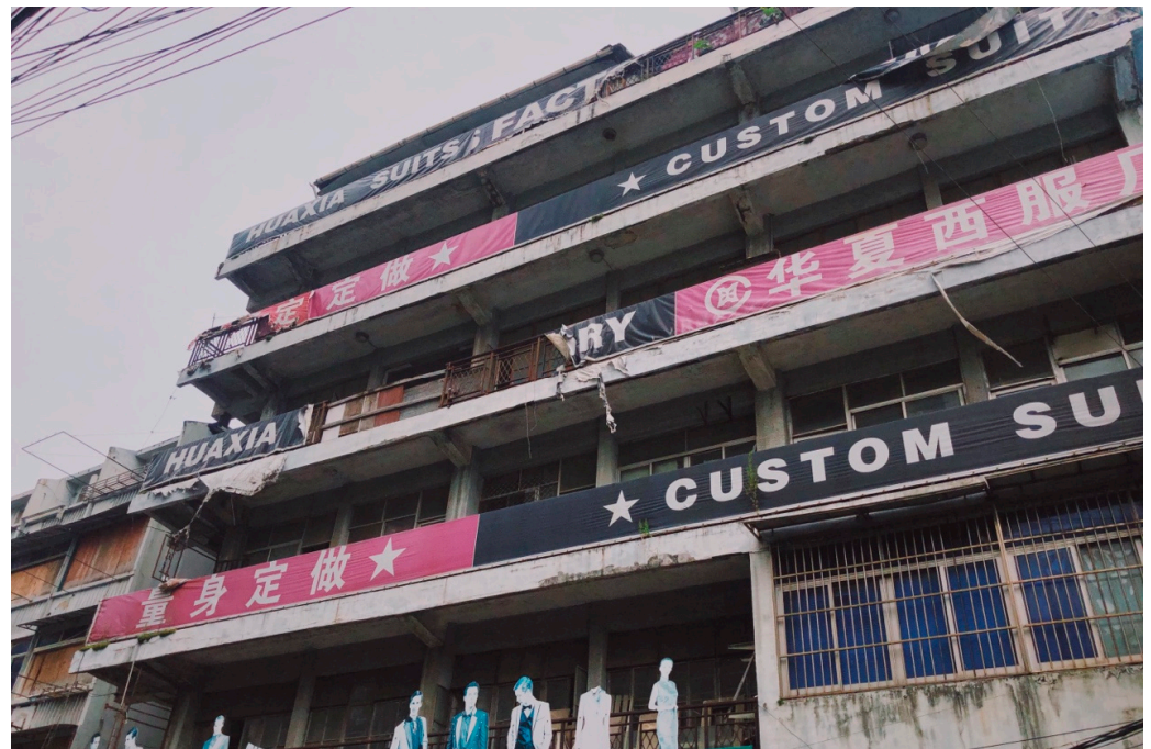
Figure 6. The once-flourishing shops in Dongjiadu are now in decline, as depicted in the image showing the façade of a custom suit store that had already experienced significant deterioration at the time the photo was taken. (source: Kaixuan Wang, 2020).
