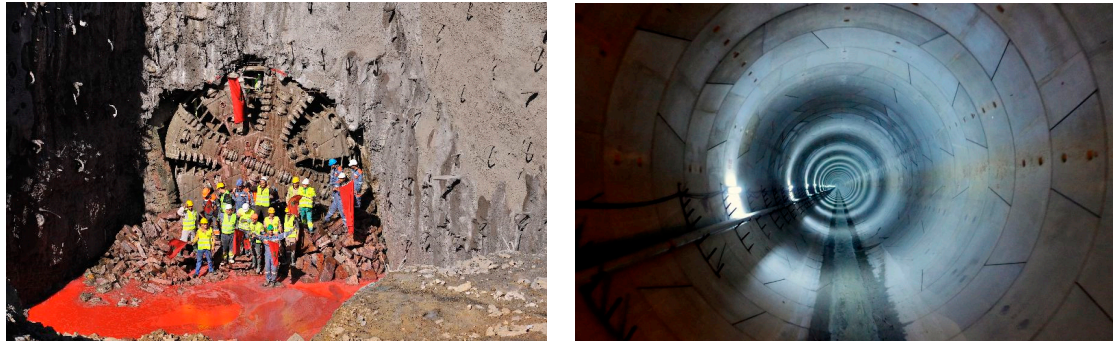
Figure 8. Construction works of the Bouskoura underground super collector (Source: Casa Amenagement).
