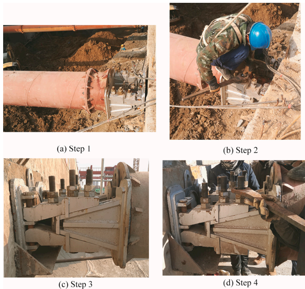
Figure 8. Field installation and demolition operation process of a BFW active joint.
