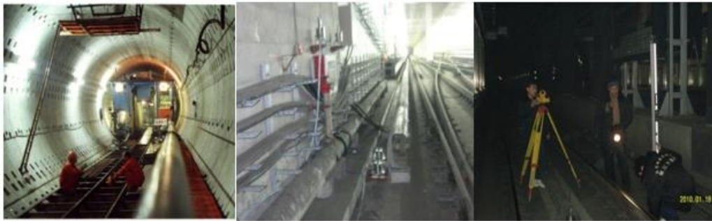
Figure 18. On-site monitoring of track deformation of the existing station.
