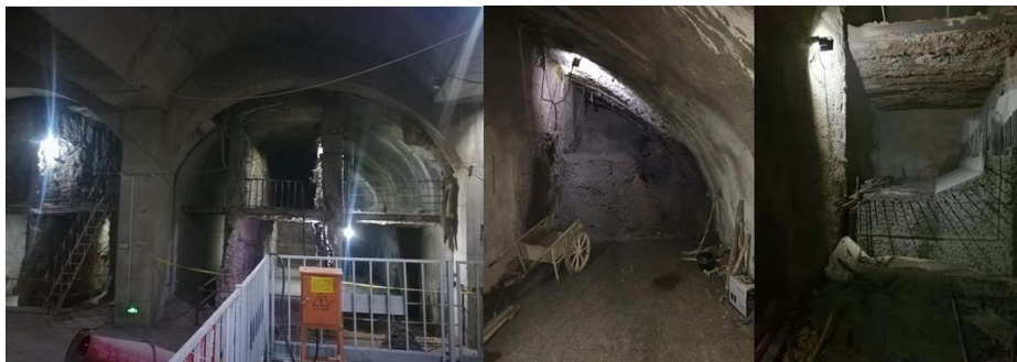
Figure 16. Excavation of multiple pilot tunnels.
