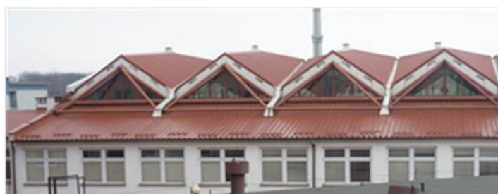
Figure 9. The external view of one elevation of the experimental hall at Rzeszow University of Technology roofed with the shell structure.
