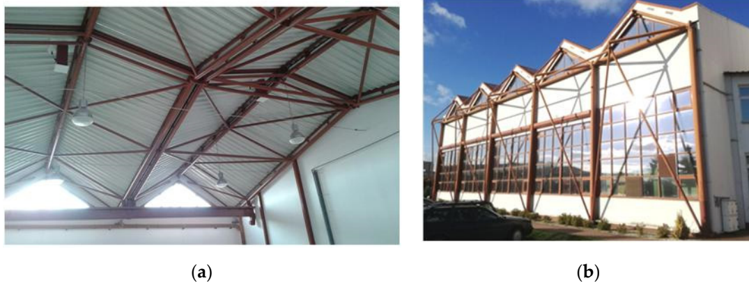
Figure 6. A symmetric shell structure roofing the experimental hall at Rzeszow University of Technology: (a) an internal view; (b) an external view.
