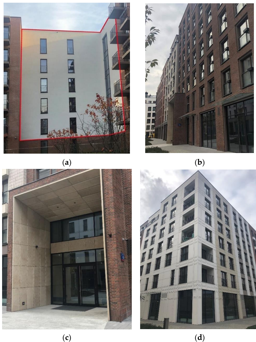
Figure 4. (a) ETICS system, (b) clinker cladding, (c) natural stone, (d) cement panels finishing [own photos].
