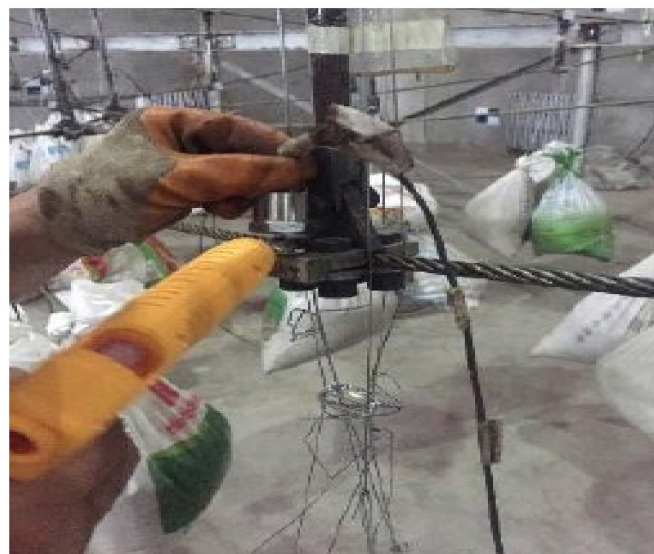
Figure 16. Maintenance of unsafe events in site construction.
