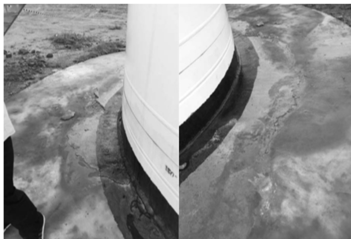
Figure 7. Foundation inspection of wind turbine No. 10.
