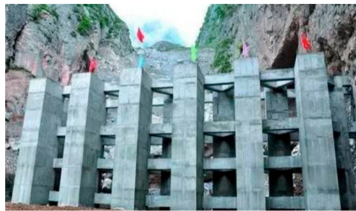
Figure 1. Typical Reinforced-Concrete Grid-type Debris Dam.
