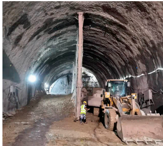
Figure 4. Temporary steel support.
