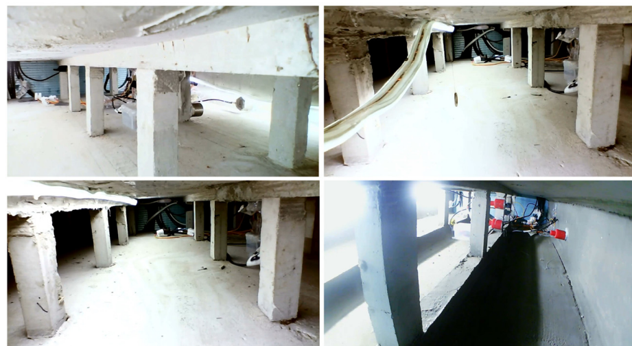
Figure 18. Inside the structure.
