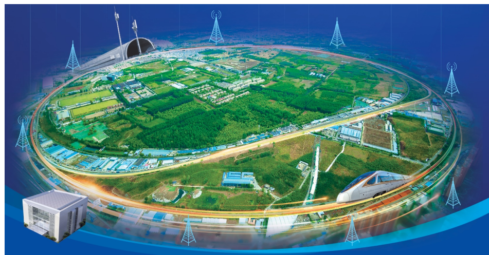
Figure 2. Test line of loop railway, National Railway Track Test Center.
