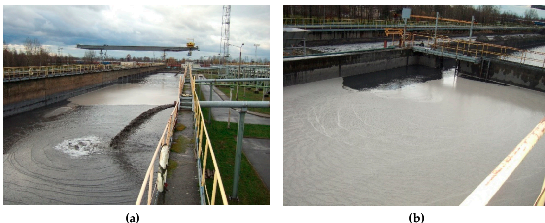
Figure 1. (a) The place of the microspheres' waste dump; (b) the microsphere on the surface of the pool.
