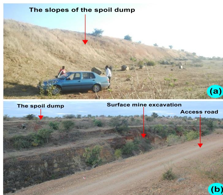
Figure 8. (a) The community facing slopes of the spoil dumps and (b) the access route and pit facing slopes of the spoil dumps at Frankie Mine.
