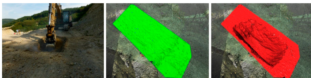
Figure 6. Collection of the large-scale sample—Probe 1. Before excavation—green left, after excavation—red right.
