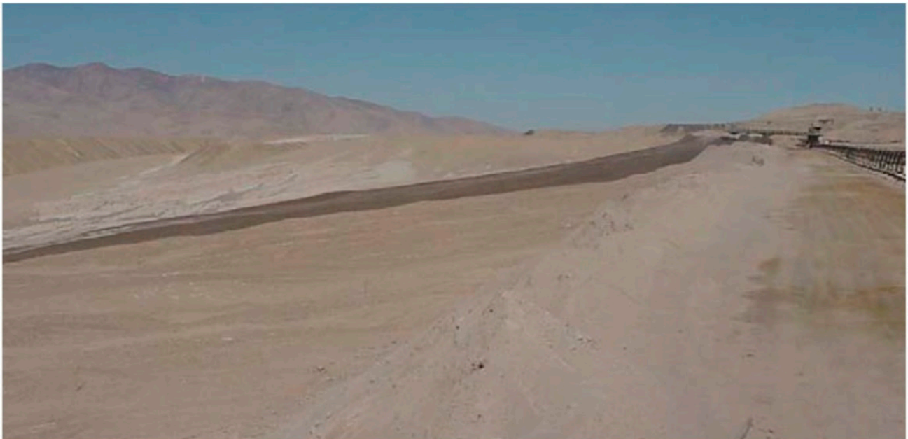
Figure 9. Mantos Blancos Disposal of Filtered Coarse Tailings with Mobile Stacker Conveyor and Tripper [12].
