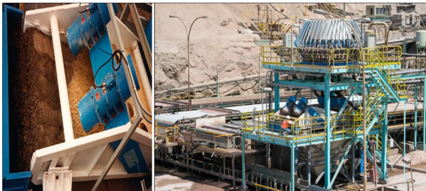
Figure 6. 1st Industrial Trial Phase of Mantos Blancos Tailings Plant 4056 mtpd: Hydrocyclone Cluster + 01 Horizontal Vibratory Dewatering Screen [40,41].
