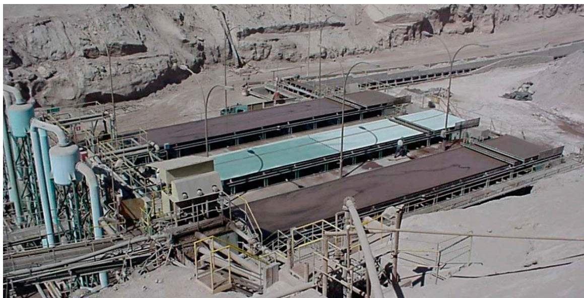
Figure 1. Tailings vacuum Belt Filters in Mantos Blancos Project [32].
