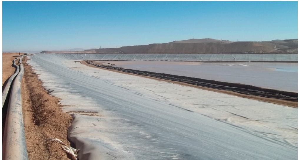
Figure 8. Mantos Blancos Disposal of Thickened Slimes in Tailings Storage Facility [39].
