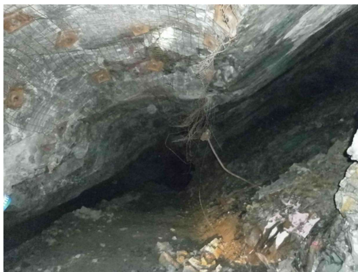
Figure 2. Development drive and low-angle stope floor after mucking by scraper. Remaining fine material in both the drive and stope floor contain liberated gold. Stope width approx. 2 m.
