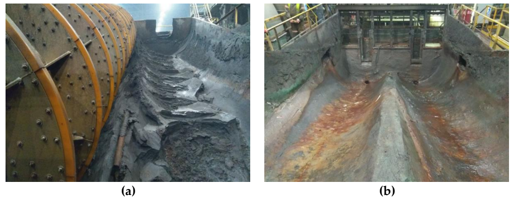
Figure 2. Preparation for anode installation: (a) view of the classifier with dismantled spiral; (b) view of the classifier with two dismantled spirals and feed removed from inside the tank.
