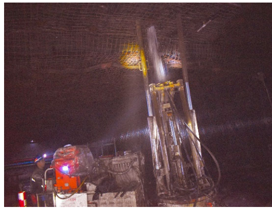
Figure 19. Large-diameter borehole drilling rig.
