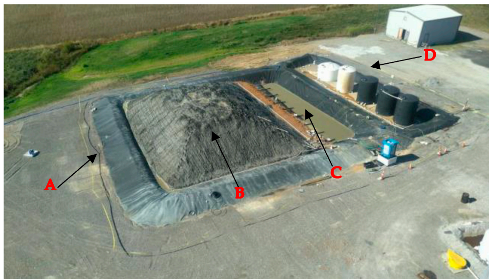
Figure 2. Aerial view of the baker seam coarse refuse heap (A) HDPE plastic liner, (B) Coarse refuse material, (C) Collection Pond, (D) Storage tanks.
