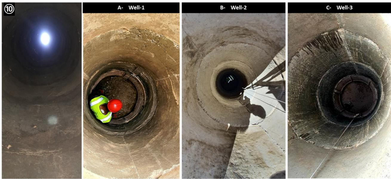
**Figure 10.** Result of excavation and final status of the three mining wells (well-1, well-2, and well-3) with different views from the bottom and from surface of the wells: ⑩ Reinforced concrete support of the wells is stable, and no signs of failure or cracking have been reported.
