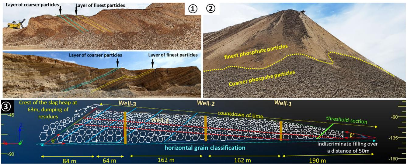
**Figure 12.** Illustration of the stockpile construction process and its evolution. ①—Artificial stratification resulting from a grain-size classification with fine particles at the top and coarse particles at the base of the screening PMWRS in ②. ③—longitudinal section showing the stockpile process construction and its evolution.
