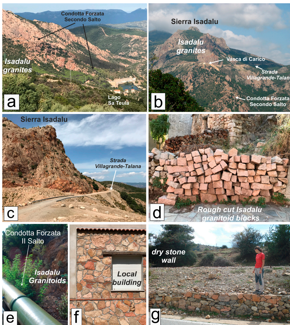
Figure 2. The Isadalu Hbl-bearing granites in anthropic environment: (a) penstocks, Sa Teula artificial basin and watermills of the Secondo Salto hydroelectric plants; (b) eastern view of Sierra Isadalu with localization of the main infrastructures; (c) the collapsing regional Villagrande Strisaili-Talana road, built over Isadalu granites; (d) Isadalu Hbl-bearing granitoid as geomaterial: rough cut blocks used for local buildings; (e) the penstocks and their relationship with Isadalu granitoids; (f,g) Isadalu granitoid blocks used for houses and dry stone walls.
