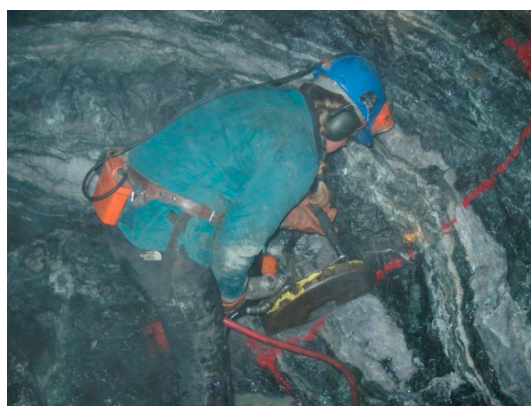
Figure 8. Diamond saw in operation during the exploration/evaluation phase.
