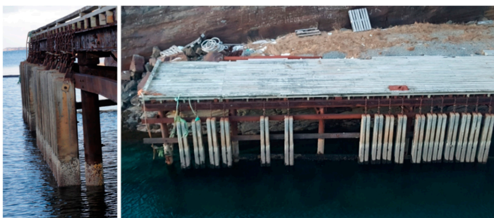
Figure 1. Picture of the concrete field station in Sandnessjøen.
