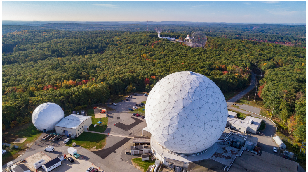
Figure 1. Aerial view of MIT Haystack Observatory. The Haystack Telescope, a dish of 37 m diameter, is located in the large radome dominating the foreground. (Used with permission, courtesy of Mark Derome).
