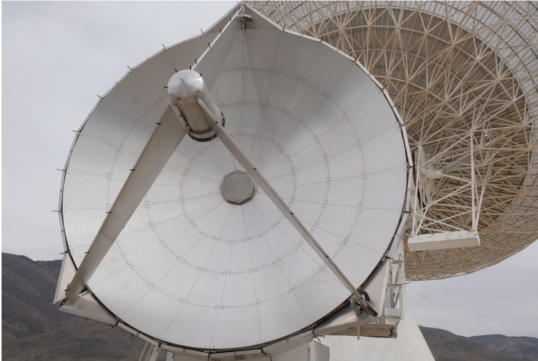
Figure 14. Photograph showing the condition of the BIMA antenna dish surface (from March 2022).
