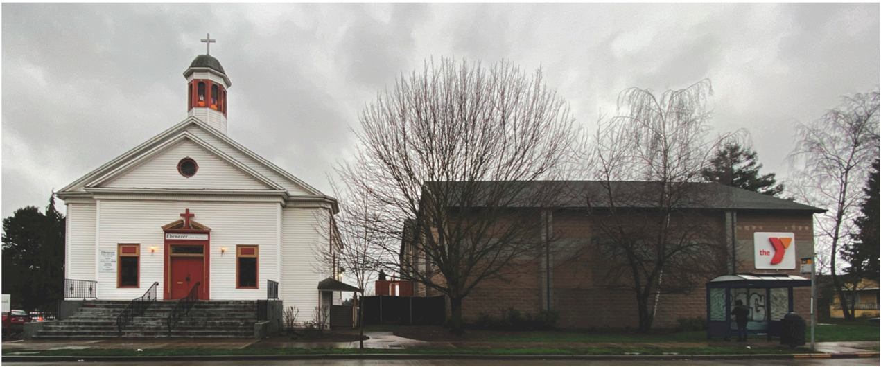
Figure 4. Existing Ebenezer AME Zion Church and the Meredith Mathews East Madison Y seen from 23rd Ave S. Source: Aubree Nichols ( Building Beloved Community , p. 60).
