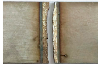
Figure 11. Joint fracture location.
