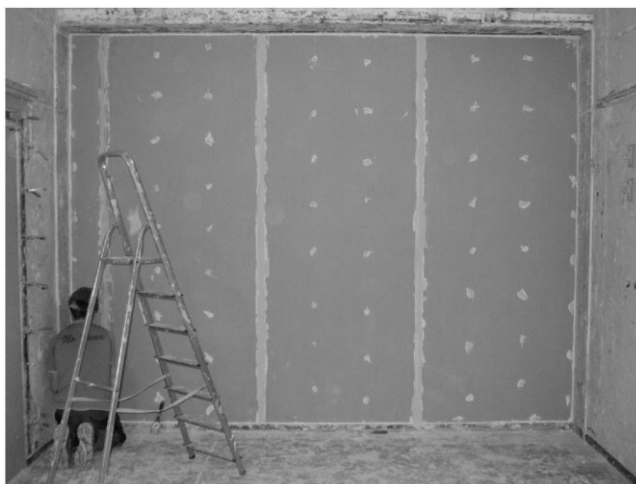
Figure 5. Mastic sealing on the metal-framed wall perimeter for the experimental test.
