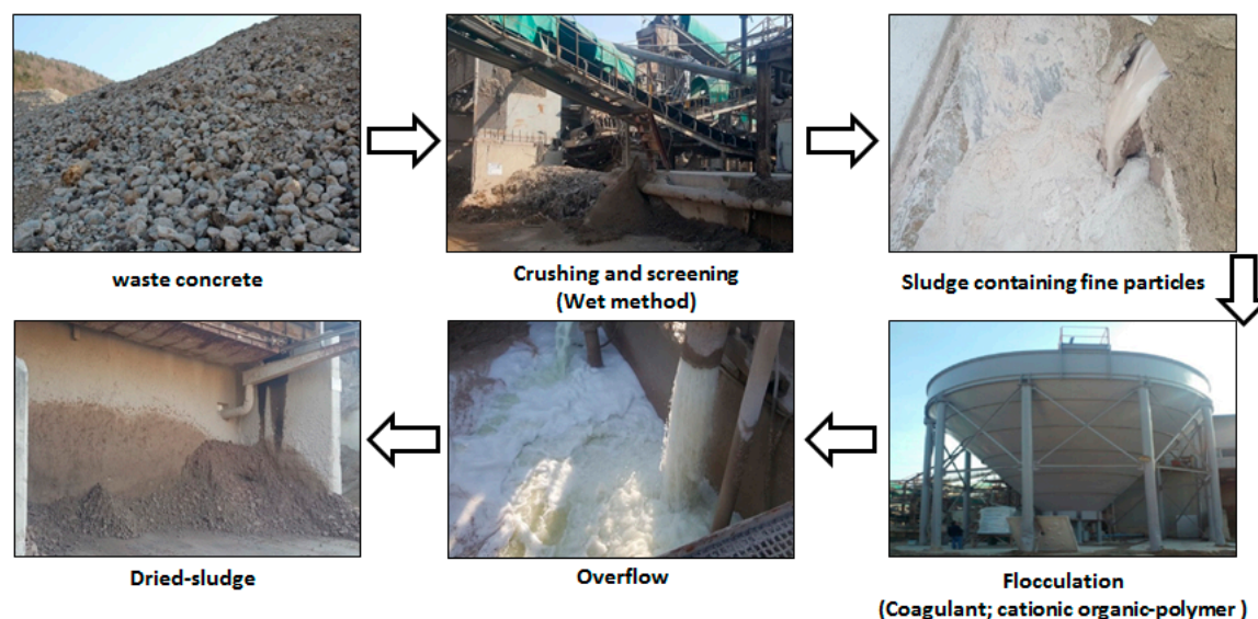
Figure 1. Photographs of a field waste concrete recycling process.
