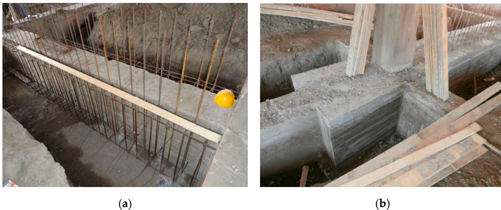
Figure 6. Footings retrofit: Steel reinforcement (a) and section enlargement (b).
