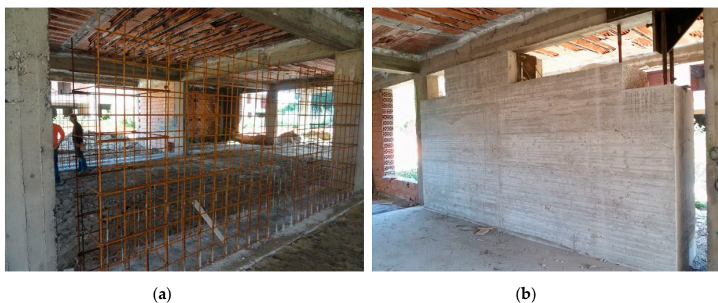
Figure 7. Reaction walls: Steel reinforcement (a) and fully casted wall (b).
