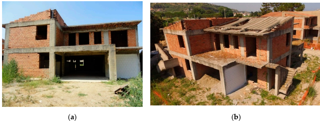
Figure 2. South (a) and north-west (b) building views.
